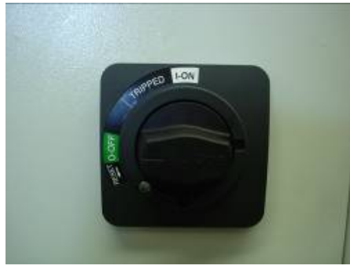
Conveyor disconnect switch
