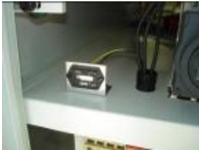
Lamp hour meter.
