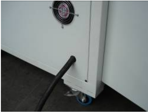
Hook-up input wires
