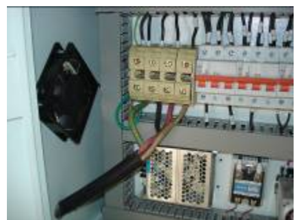
Input wire port hole
